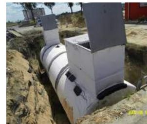
Storage tanks for PU/PIR & Pentane
